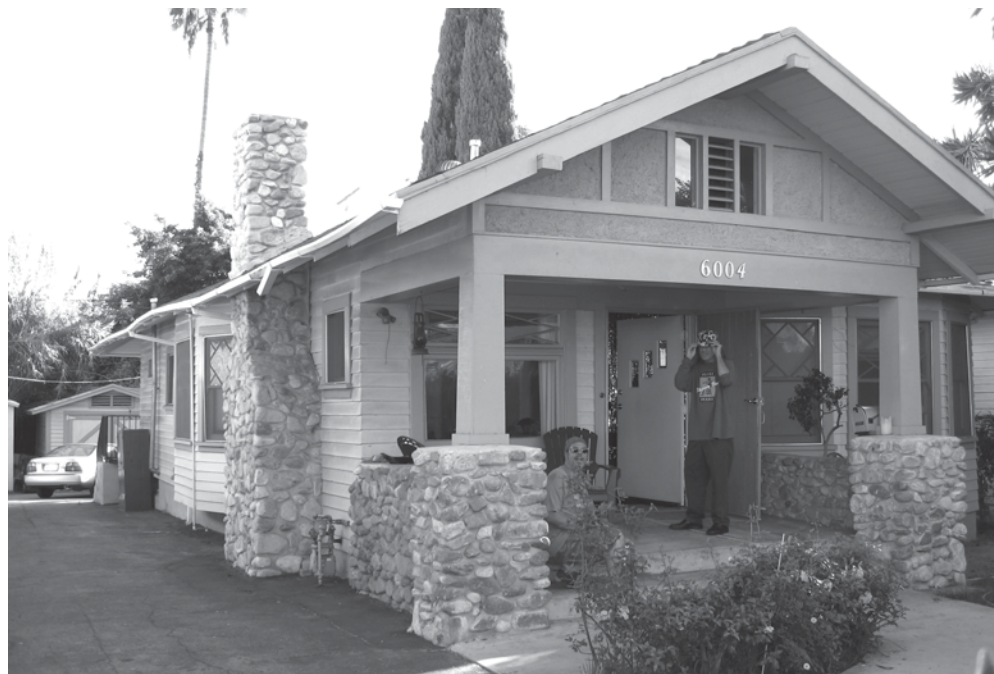
One of the Carlton Way homes endangered by illegal demolition.
