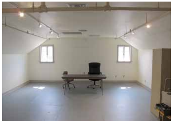
Upstairs of Barn with new enclosed ceiling.
