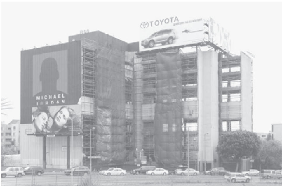
The building at 1800 Highland Avenue, under renovation
